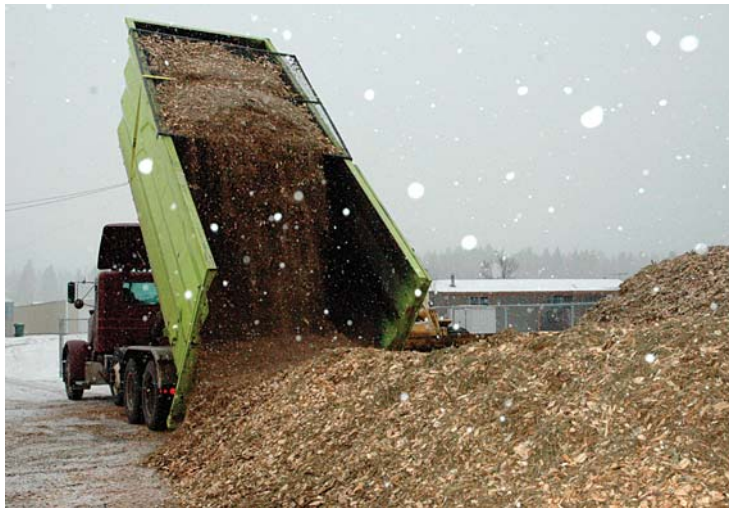
Chips being dumped at the school, will be used to fuel the wood-fiber boiler.
